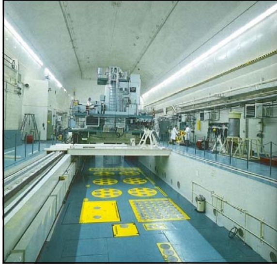
The Ågesta nuclear power plant in operation 1963-1973
